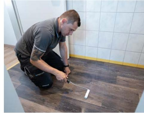
Next put a small amount of lacquer on the floor in sections and roll it thinly and quickly crosswise with a consumption of about 50 ml / m<sup>2</sup> (20 m<sup>2</sup> / liter). Make sure that the application is even in the edge and corner areas. Systematically work your way out of room. Always work wet on wet. Do not allow the lacquer edges to dry on the surface, as these would show up after drying. Please remove adhesive tape in areas of transitions immediately after sealing.
